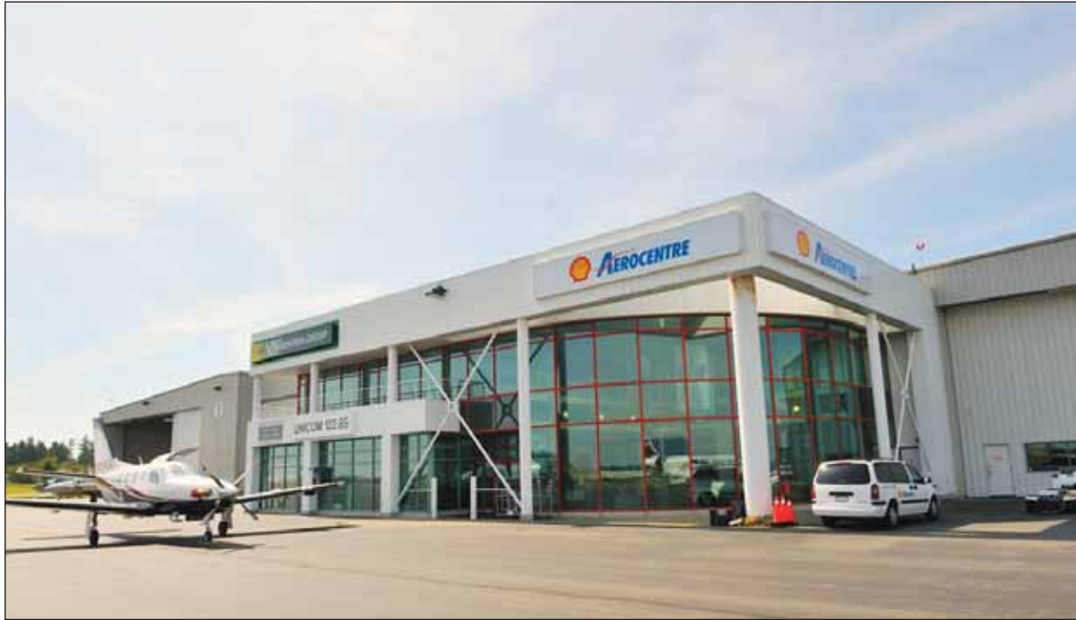
An airside view of the Shell Aerocentre
