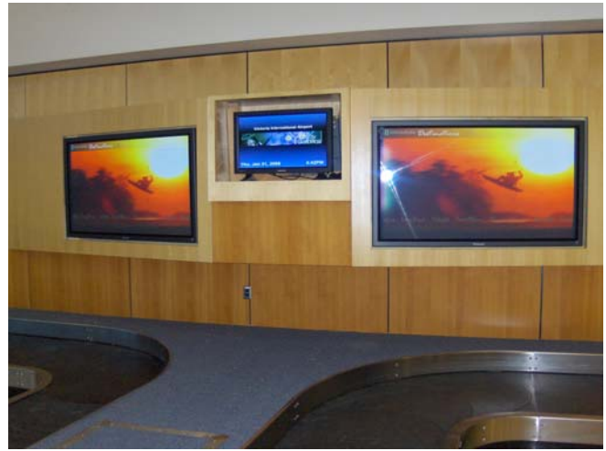
Centre Carousel – Wall with two 65” plasma displays and flight information monitor.
